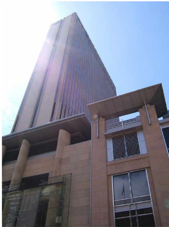
PLATE 2. The refurbished Hilton: façade and tower from George Street. Source: © Kim McNamara.
