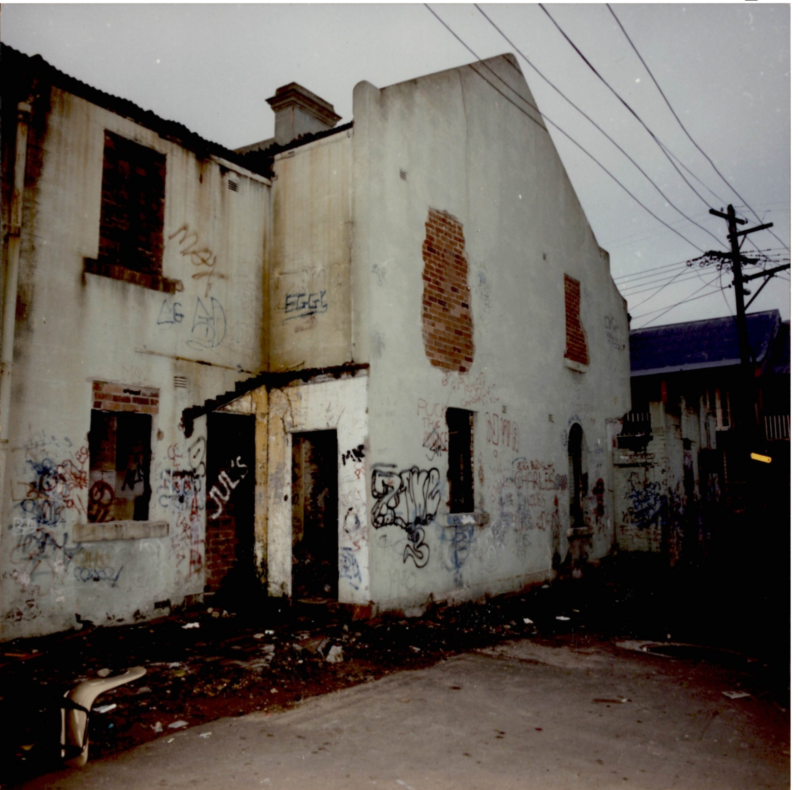
2. Side view of the exterior of No. 6 Holden Street, Redfern.
