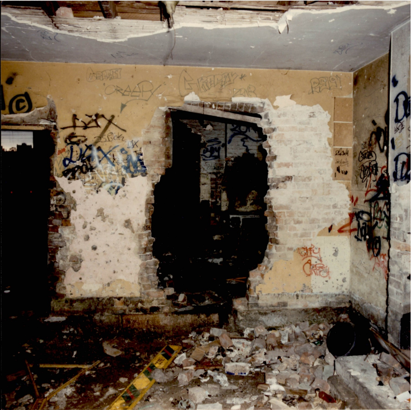
5. View of the ground floor in an easterly direction towards the railway line.
