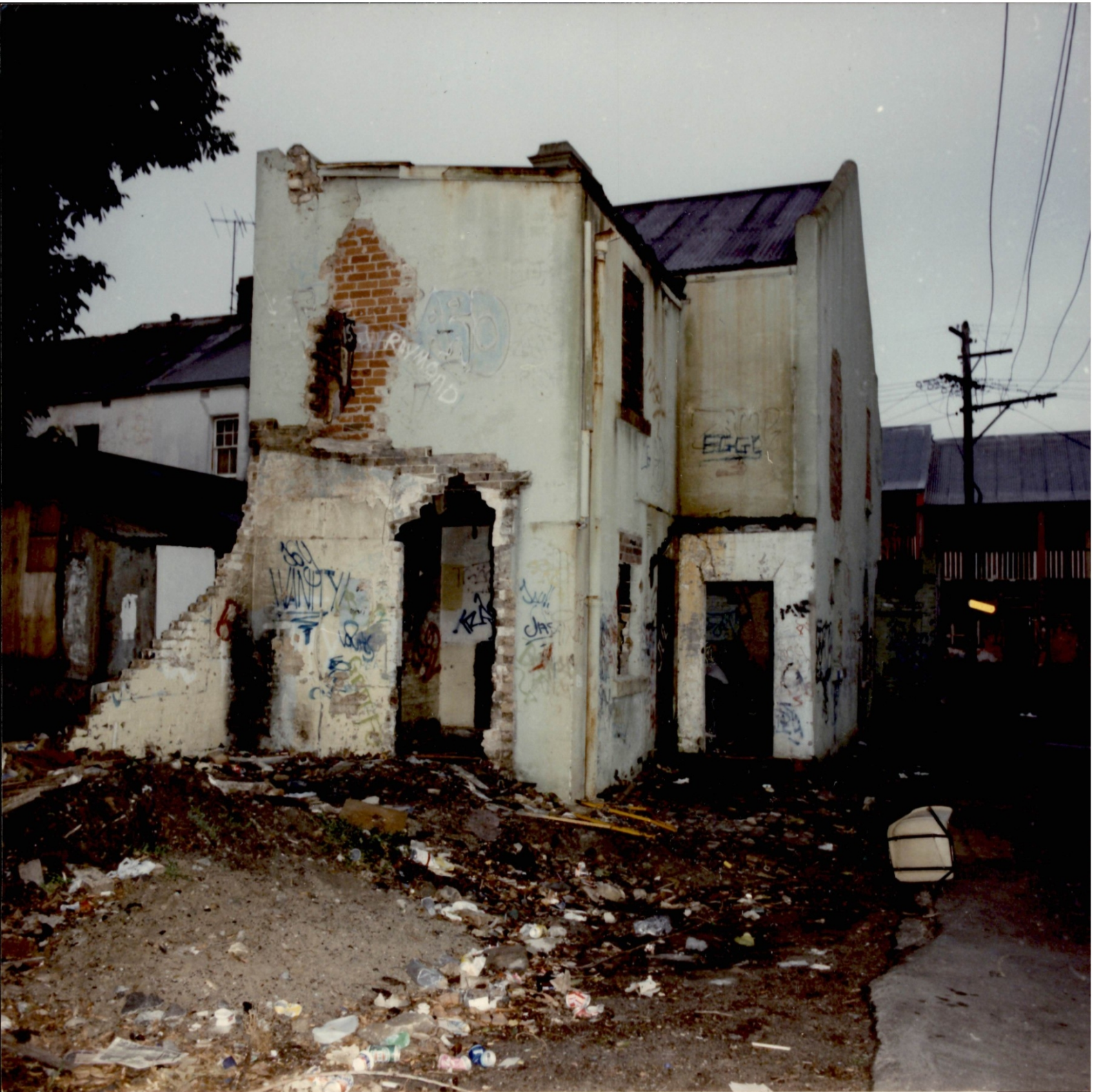
3. Rear view of the exterior of 6 Holden Street, Redfern.
