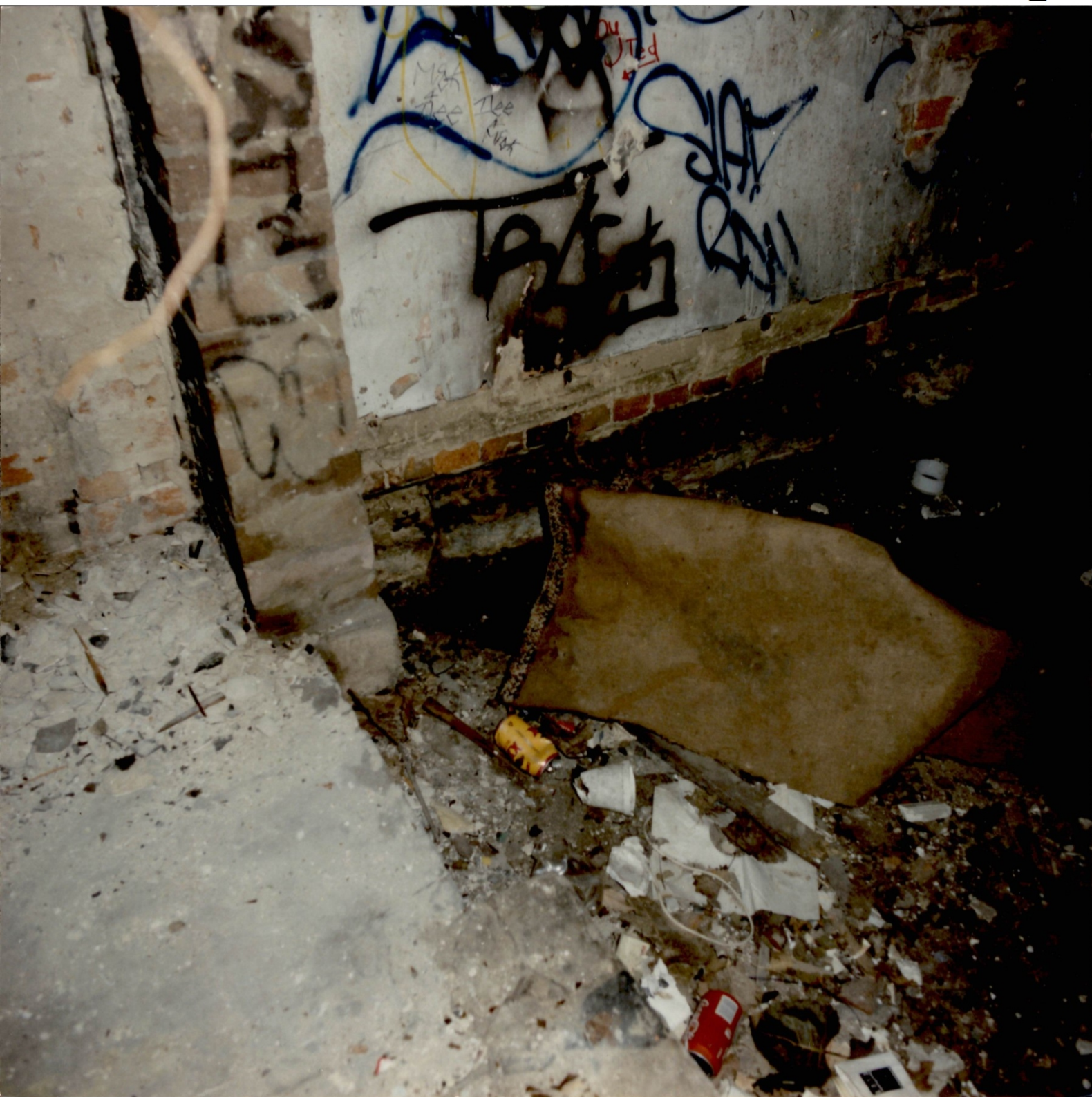
8. View of the shoes located underneath the carpet on the floor of the second room.
