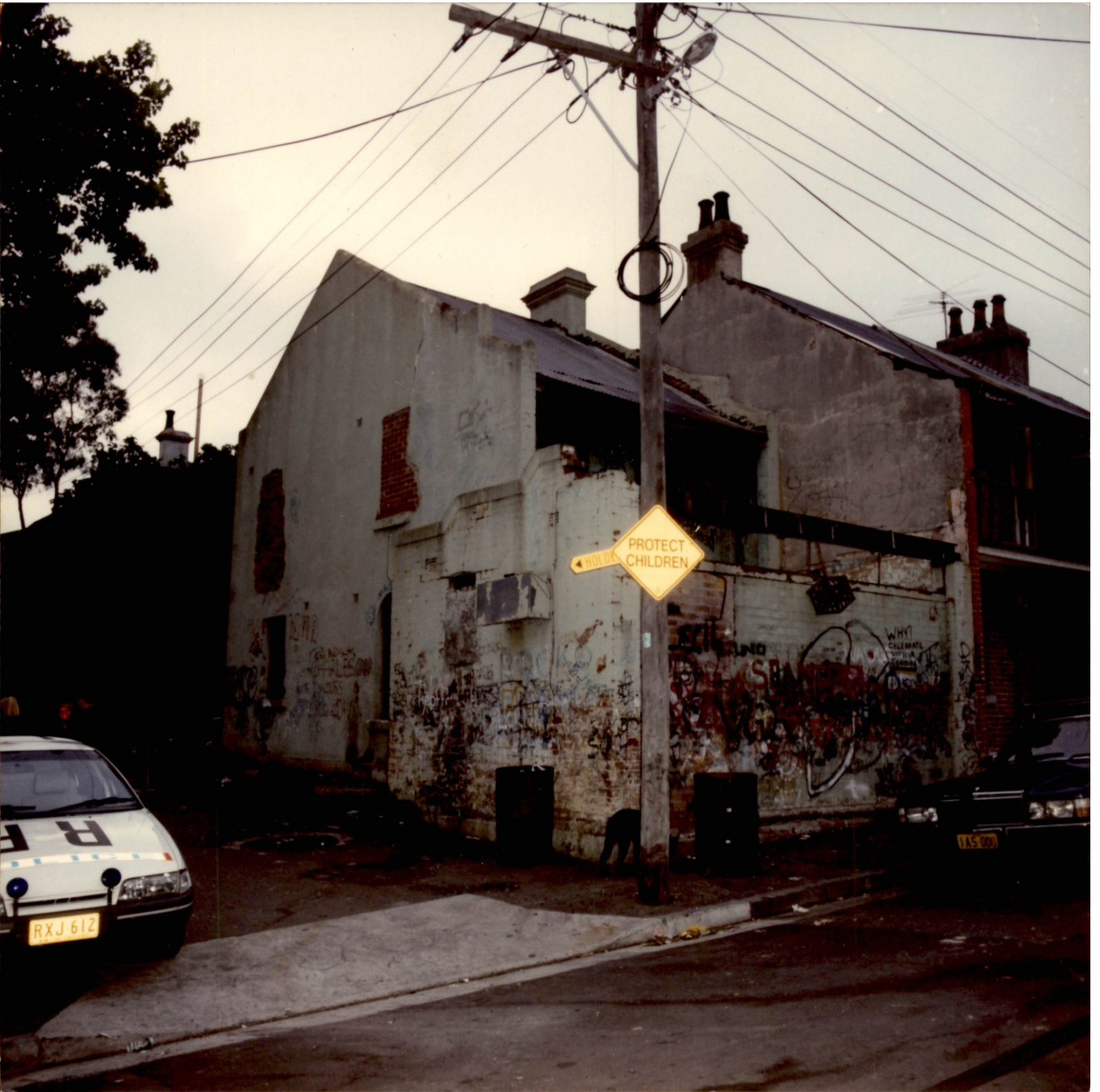
1. Front view of the exterior of 6 Holden Street, Redfern.
