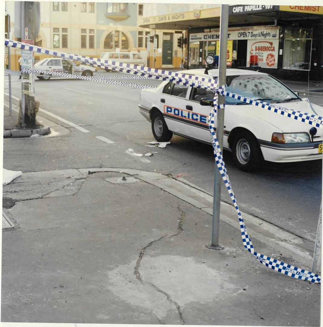
3. View east, in Campbell Street, Surry Hills.
