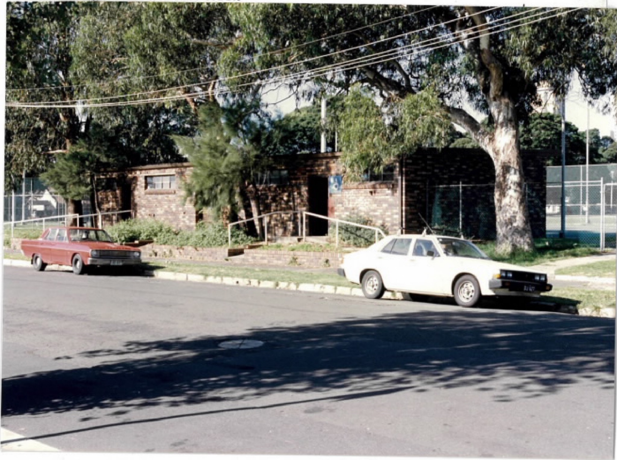
PHOTO 36. VIEW GENERALLY NORTH EAST ACROSS PARK ROAD TO AMENITIES BLOCK, ALEXANDRIA PARK.
